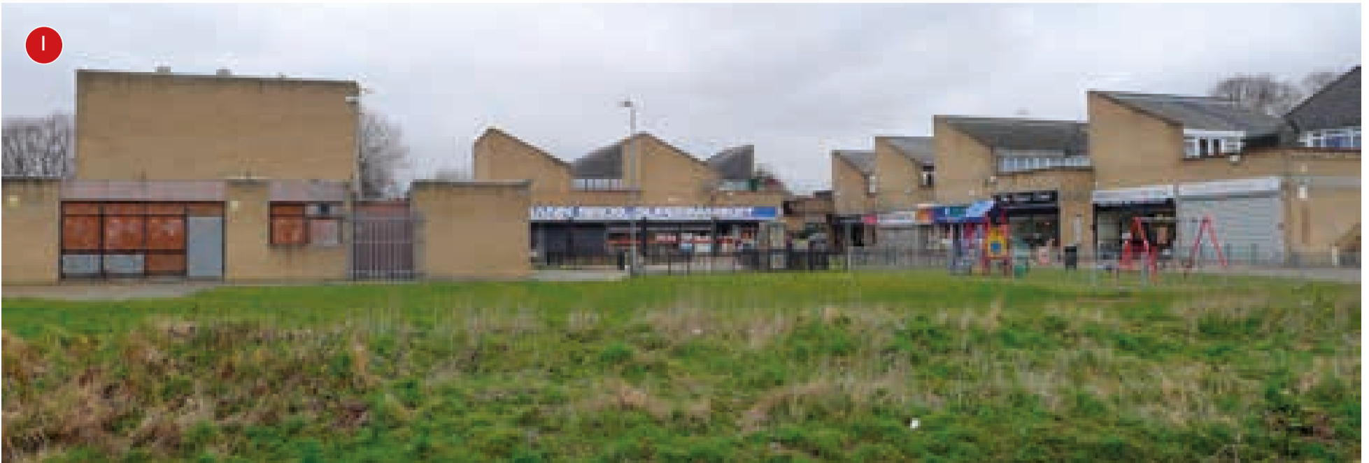
Hillhouse local shops and disused community centre (left)
