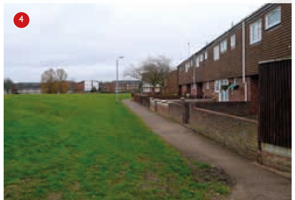
Houses fronting onto the site
